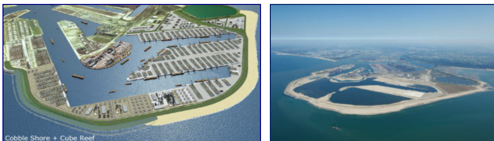
Figure 1. Maasvlakte 2 with hard sea defense designed and built (cobble shore with cube reef).
