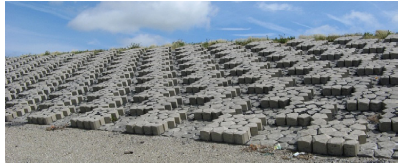
Figure 4 Basalton ® revetment placed in checkerboard pattern
