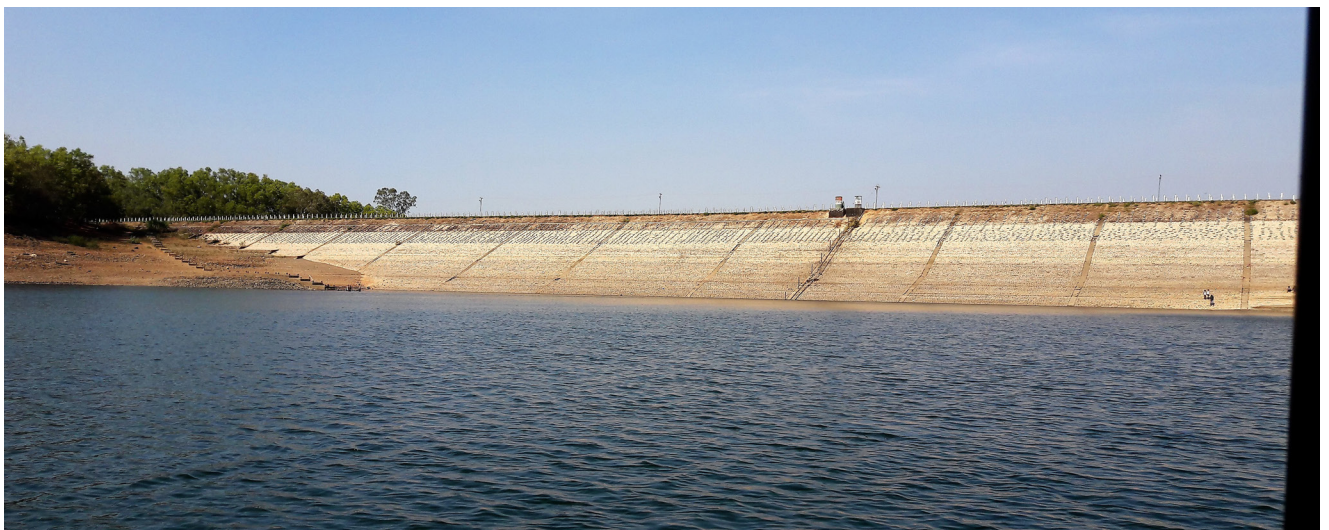
Figure 1 Bhadra embankment dam
