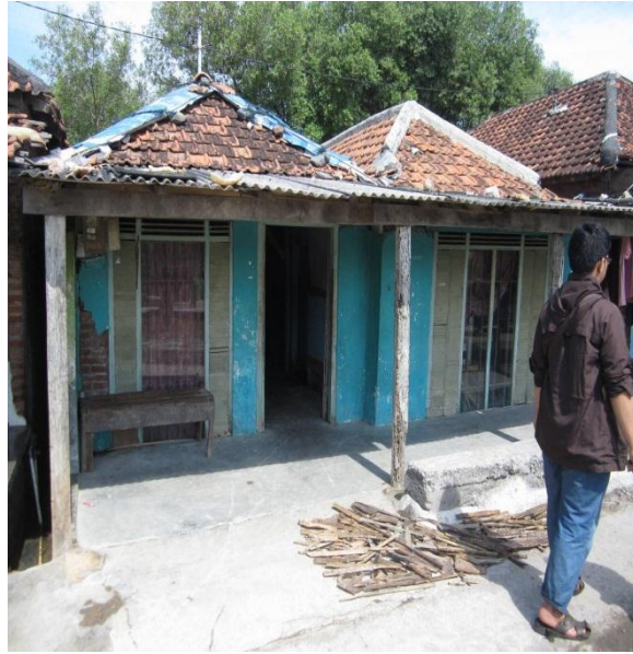
Figure 10 Houses close to the coastline in the Wonorejo part of Timbuloko. The height of the house points at the presence of subsidence (photo B.K. van Wesenbeeck).
