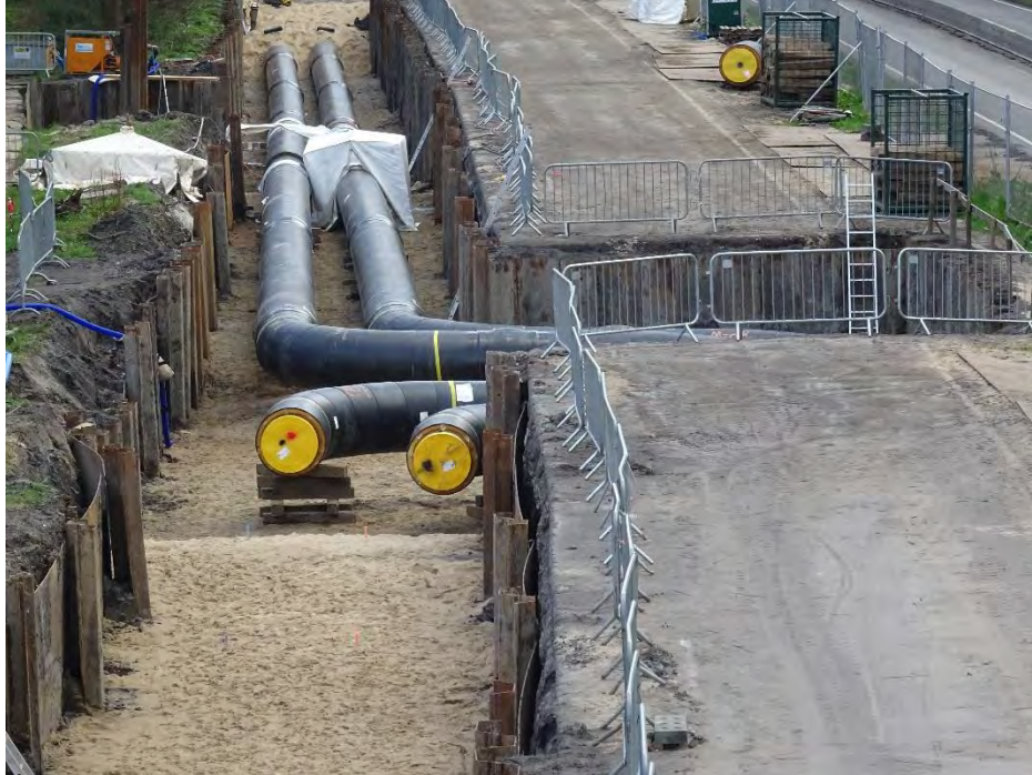
Figure 5.2: Construction of a heating network.
