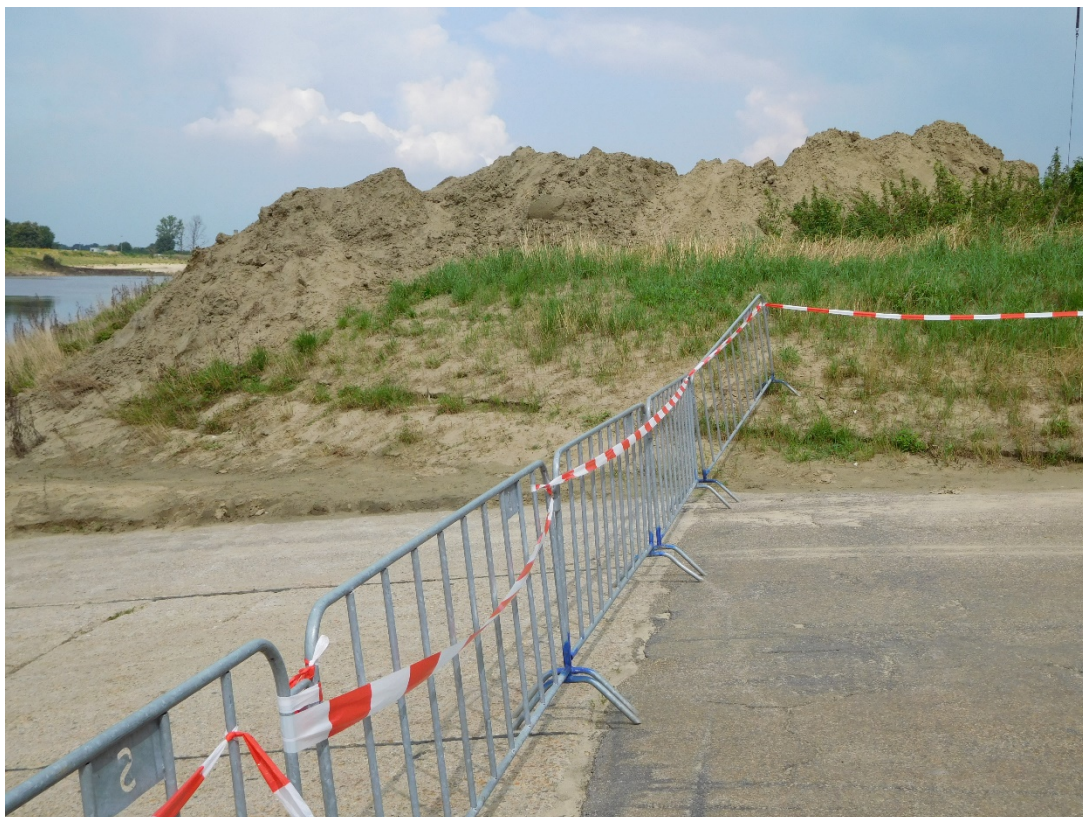
Sand deposits near the Berg aan de Maas ferry (km 38.9), still visible in the grass after being moved to the side when sand was removed from the ferry threshold.
