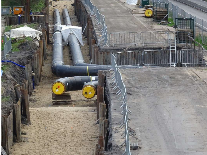
Figure 5.2: Construction of a heating network.
