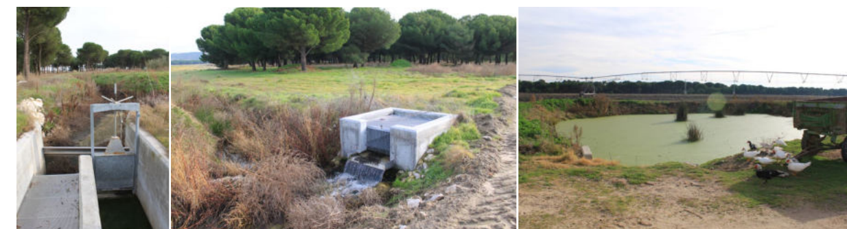
The Pedrajas-Alcazarén MAR scheme: (a) connection point where the flows from the WWTP, rooftop runoff and Pirón River diversion converge; (b) valve where the pipeline feeds the infiltration canal; and (c) previous sandpit reused as infiltration pond (source: TRAGSA).
