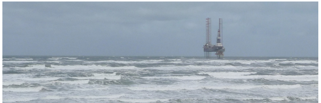
Jack-up operation in scour-sensitive area
