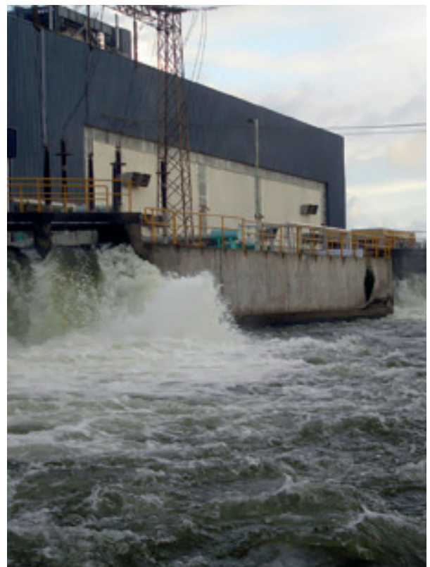
Outfall of power plant
