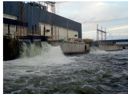
Outfall of power plant
