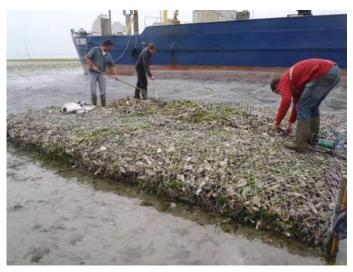
Figure 2.4 Artificial oyster reef - an example of Building with Nature to create new a habitat and mitigate wave height (source: EcoShape).
