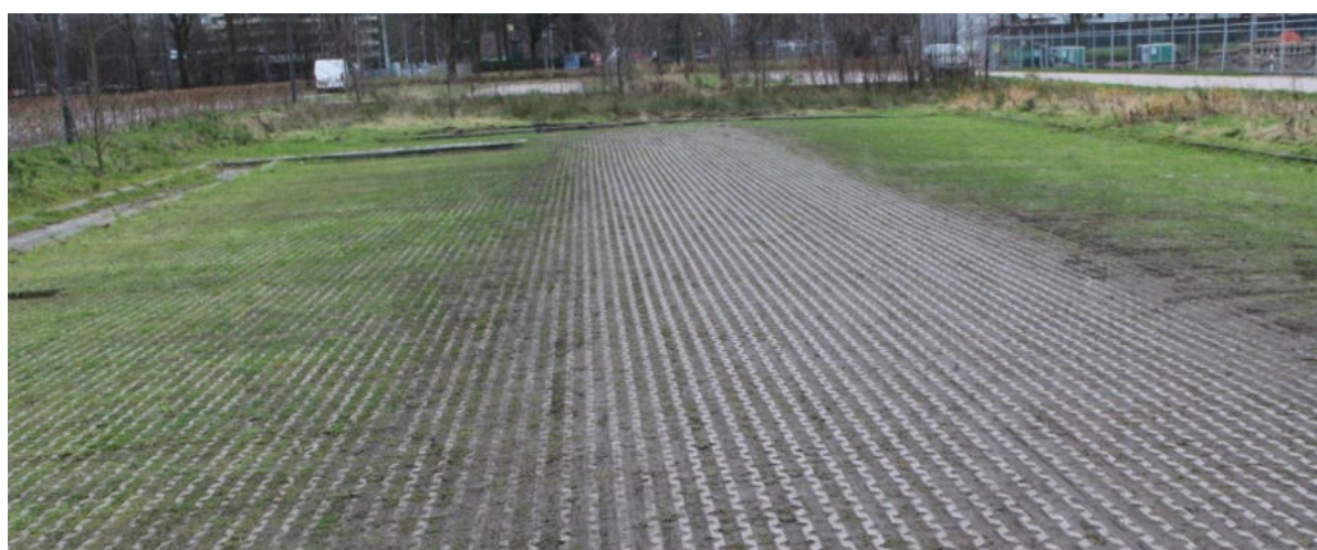
Figure 6.1: Permeable pavement can be applied to reduce the sealing grade of areas that need to be paved due their function (picture from EEA, 2016a).
