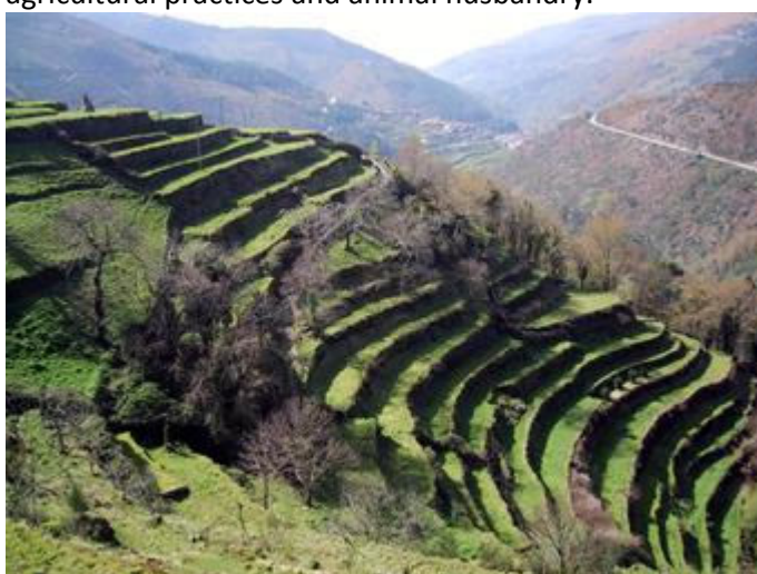
Figure 6.6: The collapsing agricultural terraces of Sistelo (Portugal).
