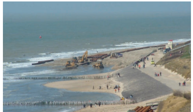
Figure 3.4: Beach nourishment in front of hard coastal defence structure near Zoutelande (Source: Zoutelande op de foto).
