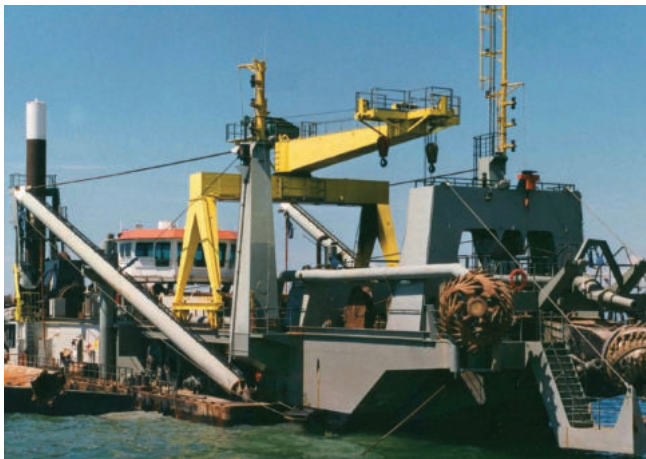
Cutter suction dredger with pipeline to the project area (Source: Van Loon Maritime Services).
