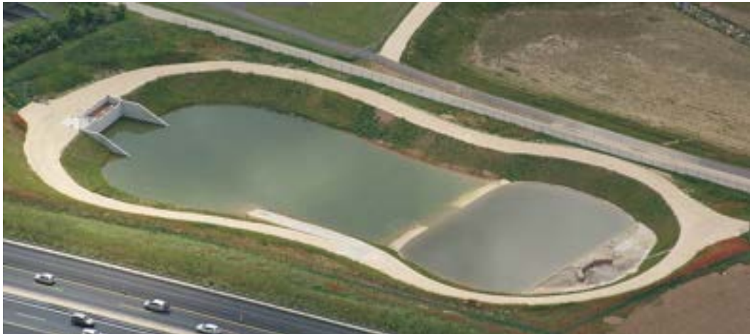
Figure 3: Rainwater retention basin Ulm
