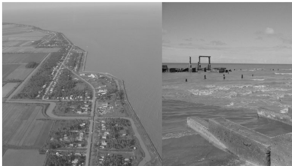
Fig. 5 Guyana mud coast around Georgetown. All mangroves have disappeared by ‘hard’ sea defences, resulting in severe coastal erosion, as shown from the abandoned sluice systems
