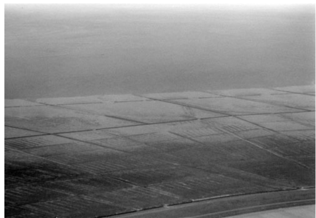
Fig. 12 Example of salt marsh works along the Wadden Sea (The Netherlands) – such salt marsh works, consisting of permeable groins made of willow twigs, have been deployed for many centuries, reclaiming substantial areas from the sea
