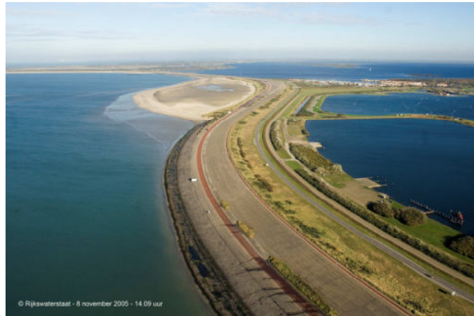
Figure 1. The Brouwersdam a closure dam with an asphalt dike revetment (source: Rijkswaterstaat, www.kustfoto.nl )
